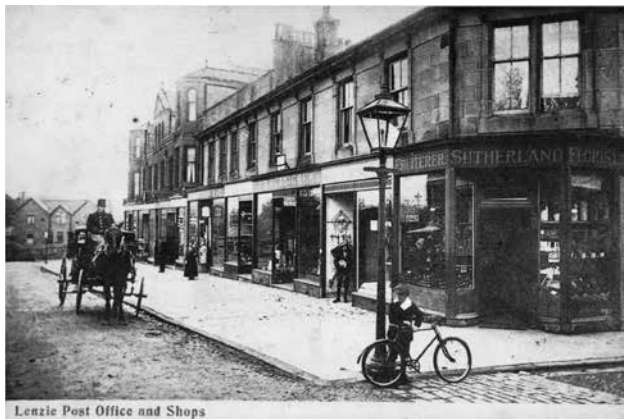
Lenzie Post Office and Shops
